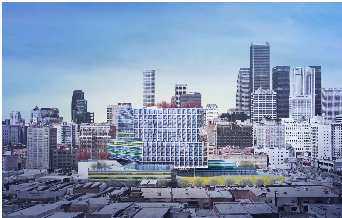
Figure 3. The Southern California Flower Market, 755 Wall Street, Los Angeles, Ca. Mixed-use, 323 apartments over office, parking, retail, restaurants and a working flower market. 10% moderate-income units. 84 units/acre. Architect: Brooks + Scarpa Developer: The Southern California Flower Market. Obtaining entitlements to allow housing in the industrial zone, the new ReCode LA zoning update is anticipated to allow this type of project by-right.
