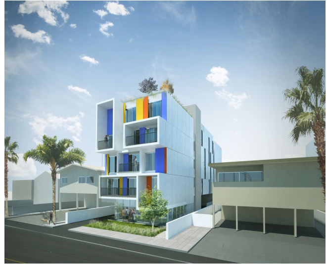
Figure 5. NEST Toolkit, awarded $1mil grant in 2019 for 'thinking outside the box to address homelessness throughout LA County'. A 'kit-of-parts' that can be built off-site and assembled quickly. Designer/Architect: Brooks + Scarpa. Team members: PlantPrefab and Community Corporation of Santa Monica. Tailoring the prefab custom home building industry to permanent supportive housing development for temporary and permanent housing at all scales and types on lot sizes from the typical suburban lot size of 50' x 150' and up.
