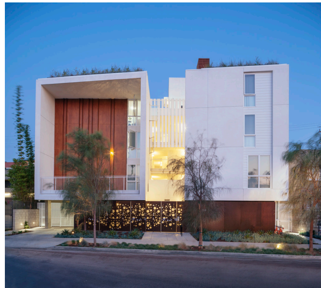
Figure 1. Gateway Apartments, 13368 Beach Ave, Venice, Ca. 21 one-bedroom apartment units. 100% affordable housing for homeless adults. 111 units/acre. LEED Platinum. Architect: Brooks + Scarpa Developer: Venice Community Housing Corporation. Utilized the local density bonus ordinance (# 179681) and the State of California's low-income housing tax credit program.
